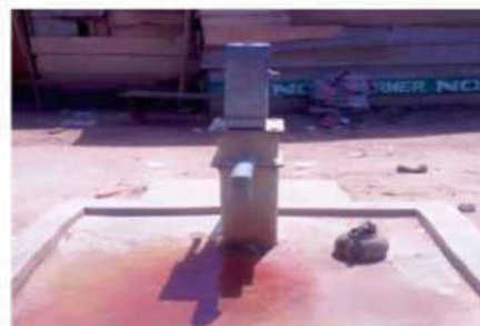
Non-functional Hand Pump Borehole @ Ikunrin Market
