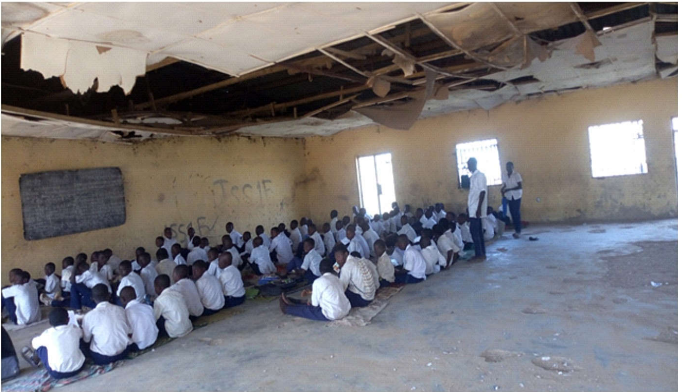
Government Secondary School, Kargi Road, Tudun Wada
